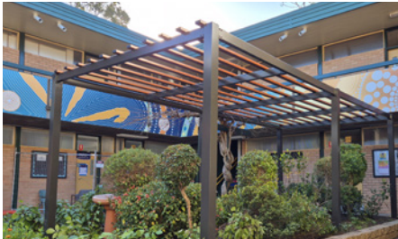
4x2m Manchester Pergola (Custom Configuration)
